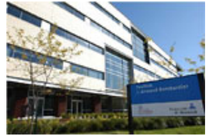
Our facilities at the J.-A.-Bombardier Pavillion
